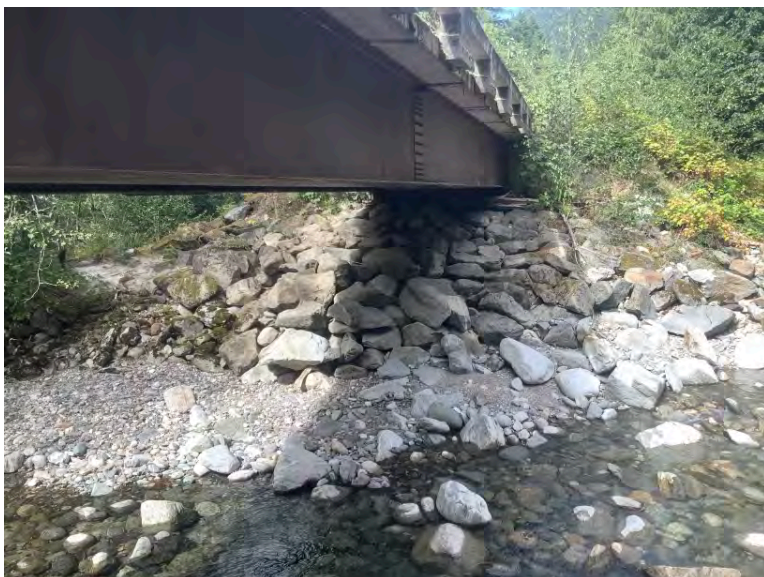
Right Bank Abutment when facing downstream
