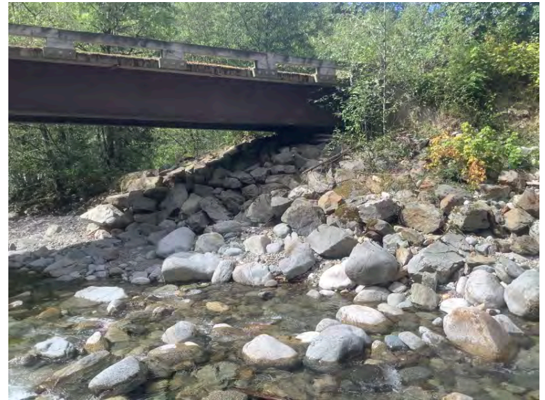
Right Bank Abutment when facing downstream
