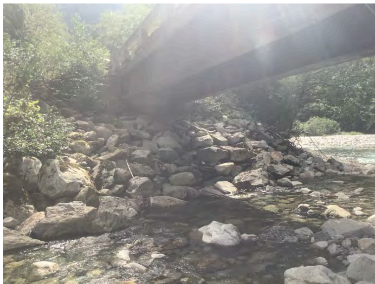
Left Bank Abutment when facing downstream
